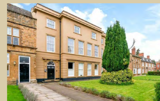
Mercia House, Banbury Developed by Walker Graham Architects | PC 2016
