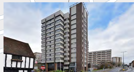
Miller Heights. Former office building converted to 100 residential apartments in 2015
